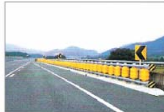
Newly constructed National Road between Sungjoo and Wyeqwan
